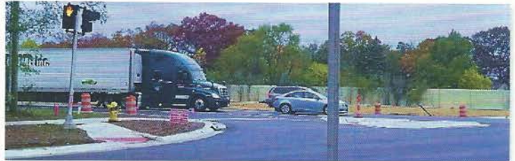
Ypsilanti Twp., Washtenaw County, and Van Buren Twp. US-12 Design-Build, Wayne County
